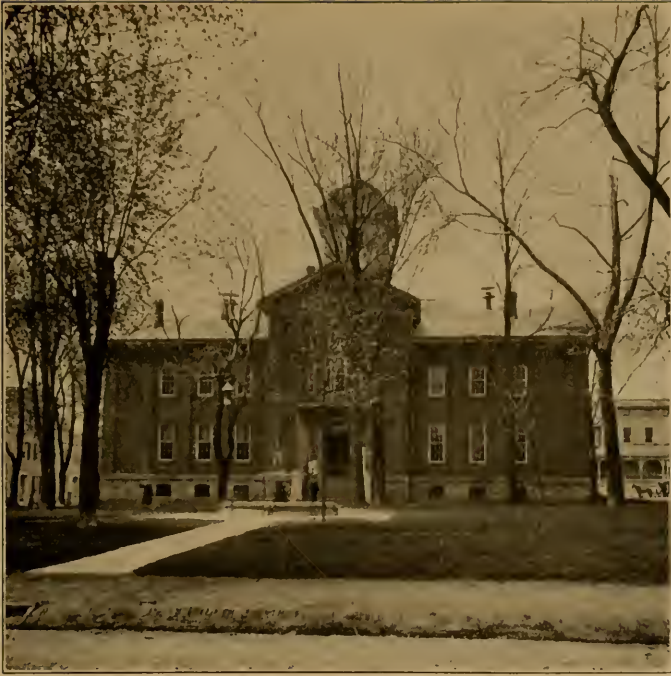
COURT HOUSE AT FREDERICK.
